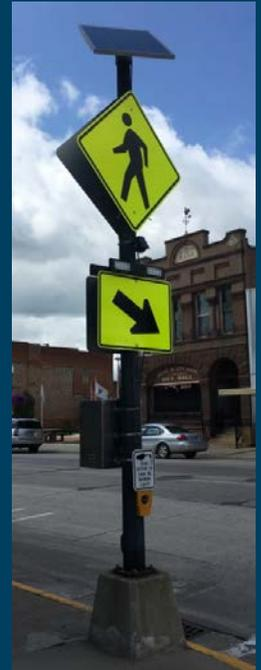
Push button and motion activated, LED-enhanced crossing system in Sleepy Eye, MN (1<sup>st</sup> Ave / HWY 14)
